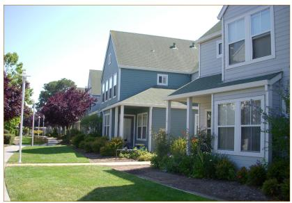
Developer MidPen Housing Corp. Property Management MidPen Property Management Corp. **Development Type** New construction: two- and three-story townhouse-style apartments **Construction Type** Wood frame with composition shingle roofs Site Area: 4.9 acres Density: 20 units / acre Parking Ratio: 1.9:1 - 186 spaces **Development Profile** Type No.
